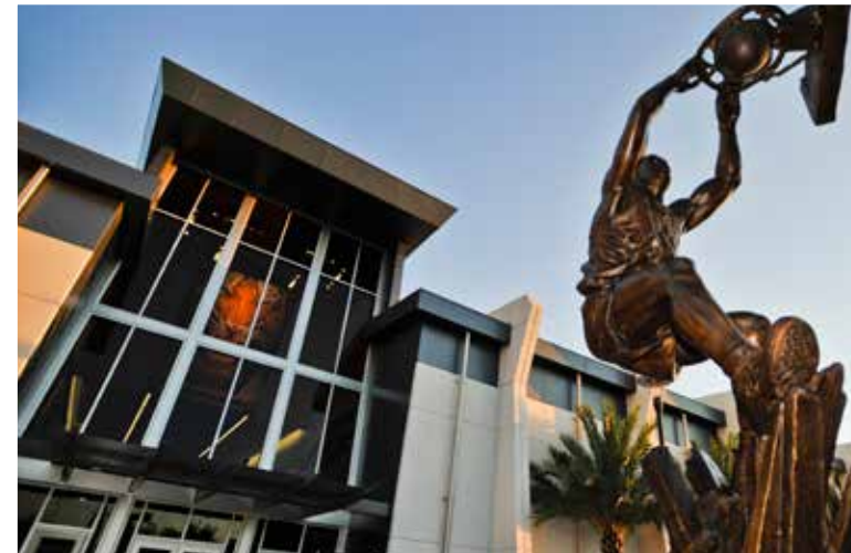
LSU Basketball Practice Facility Louisiana State University, Baton Rouge, LA
